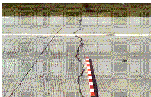
fissure transversale
